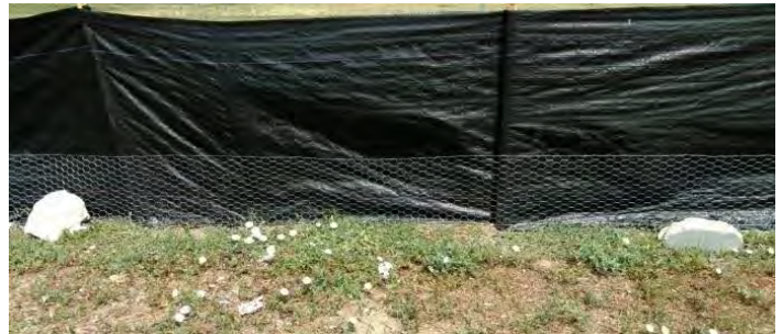
Modification: Using 2 foot-wide one-inch netting poultry wire, lip one foot vertically and use a staple gun to attach to wood posts. Anchor horizontal piece to ground with 6-inch pins.
