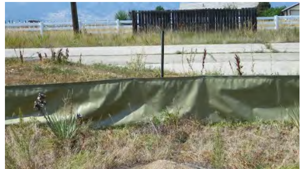
Flawed vinyl barrier installation
