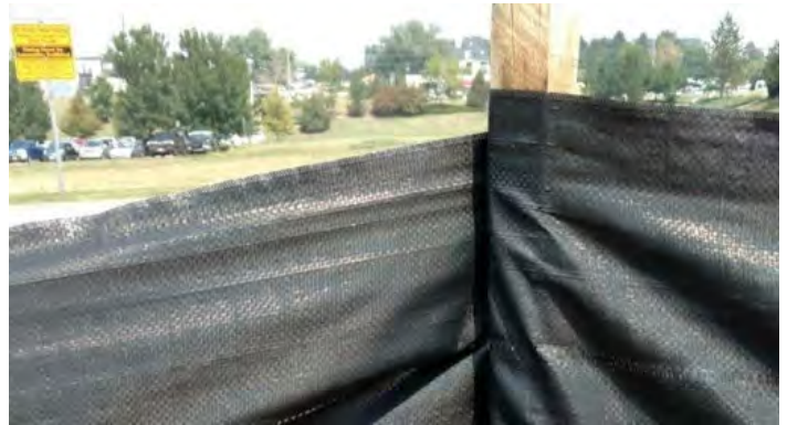
Modification: Twist fabric around stake for longevity
