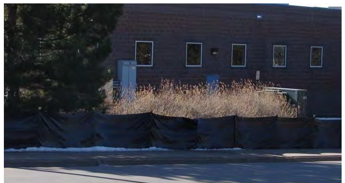
Silt fence used for pending construction.
