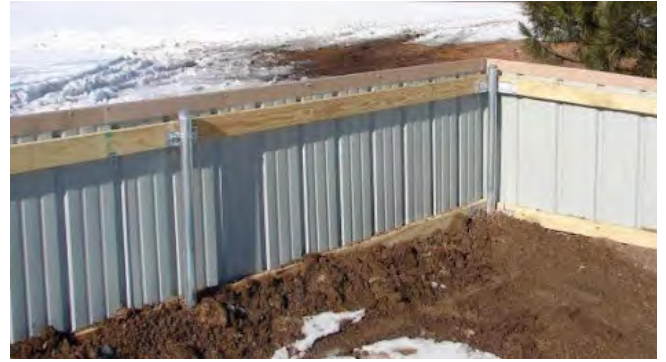
Prairie dog side of barrier. Note safe caps on metal posts and elongated cap along top of metal fencing.
