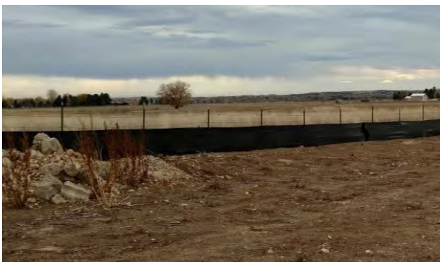
Silt fence used in large field.
