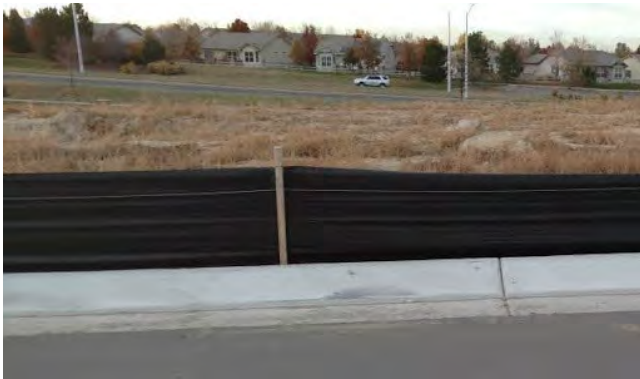
Silt fence with stakes and staples exposed.
