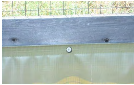
Screw and washer through grommet
