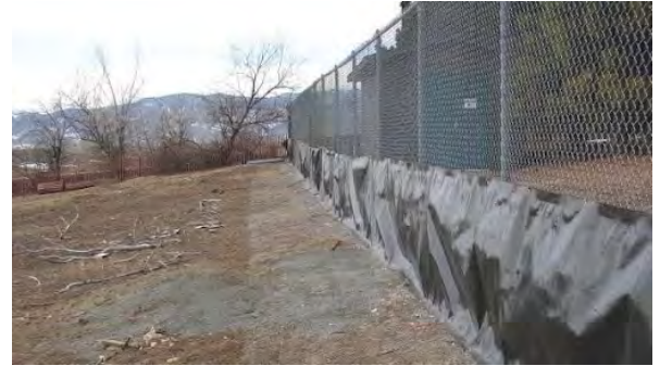
Modified existing chain-link fence to inhibit movement back into park (prairie dog side).
