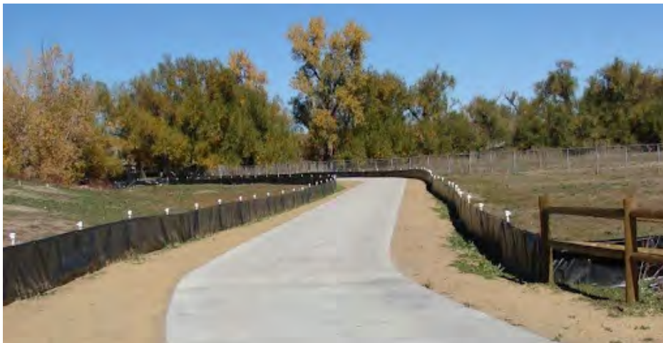
Temporary vinyl barrier used during construction project.
